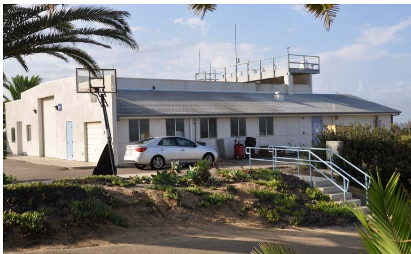
Figure 58. Commander Everett added the north wing machine shop lean-to addition (behind car) to Building F-36 in 1991, which was later expanded westward (to right of windows) as part of the contracted south-wing addition to the building (extreme left) in 2010.
