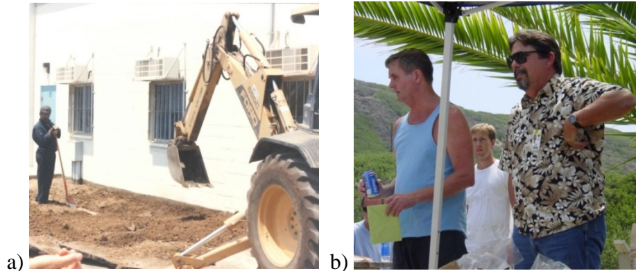
Figure 61. a) A 6-foot-wide concrete apron was added around F-36 to provide more complex pathways for testing the MDARS-Interior robot. b) Commander Bart Everett (left) delivers a heartfelt thank-you speech for Seaside Facilities Manager Tom Gaydos during the latter's potluck retirement picnic at the volleyball court.
