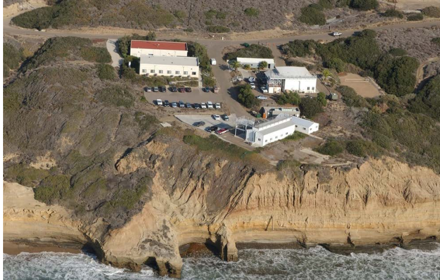
Figure 63. Newly constructed Buildings 622 (grey roof) and 624 (red roof) are shown at upper left in this aerial view of the growing unmanned systems campus overlooking the Pacific Ocean on Woodward Road looking east, circa 1994. Note sand volleyball court just to the south at center right.
